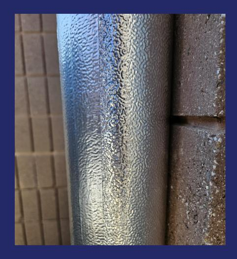
Water-Tight Butt Joints and Lap Seams are your best Defense to Prevent Moisture Infiltration. Note: All Corrosion starts with Moisture
